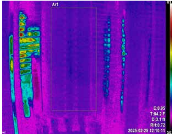
Infrared thermal image
