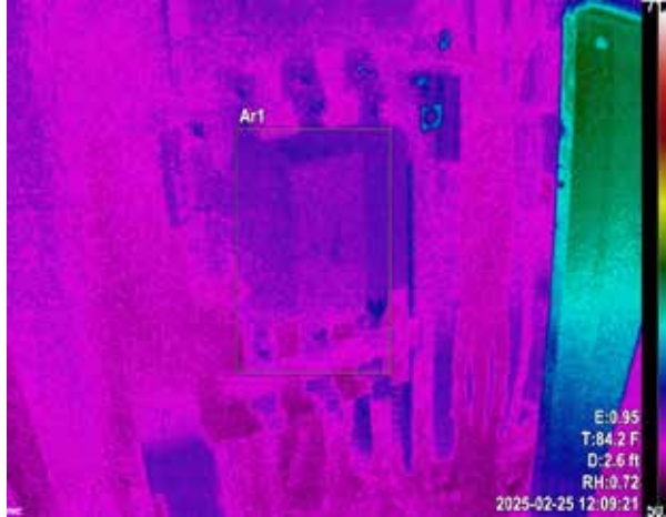
Infrared thermal image
