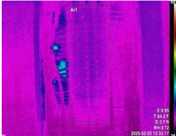
Infrared thermal image
